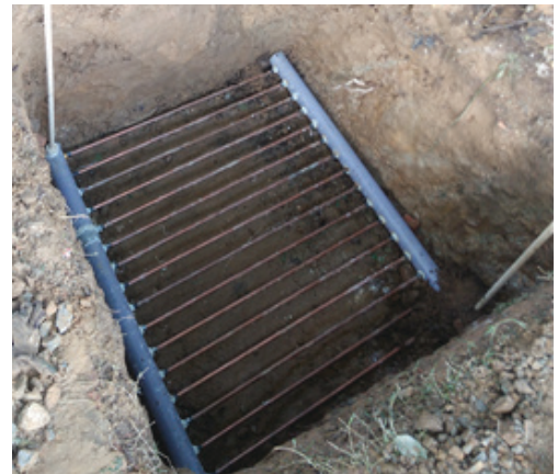
Fig: Pictorial Representation of Earth Air Tunnel
