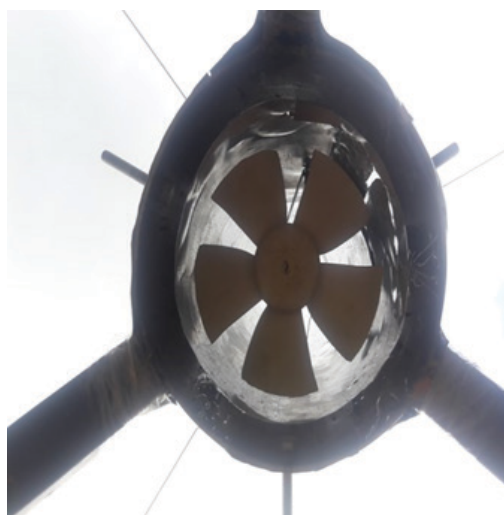
Fig: Turbine Connected to shaft
